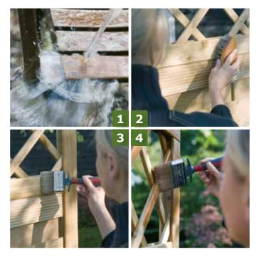
Exterior Oil is used for the basic treatment and maintenance of wooden facades and fences. The oil provides the wood with a hardwearing surface and a golden shade and enhances the natural wood grain. All variations are equipped with UV-protection.
